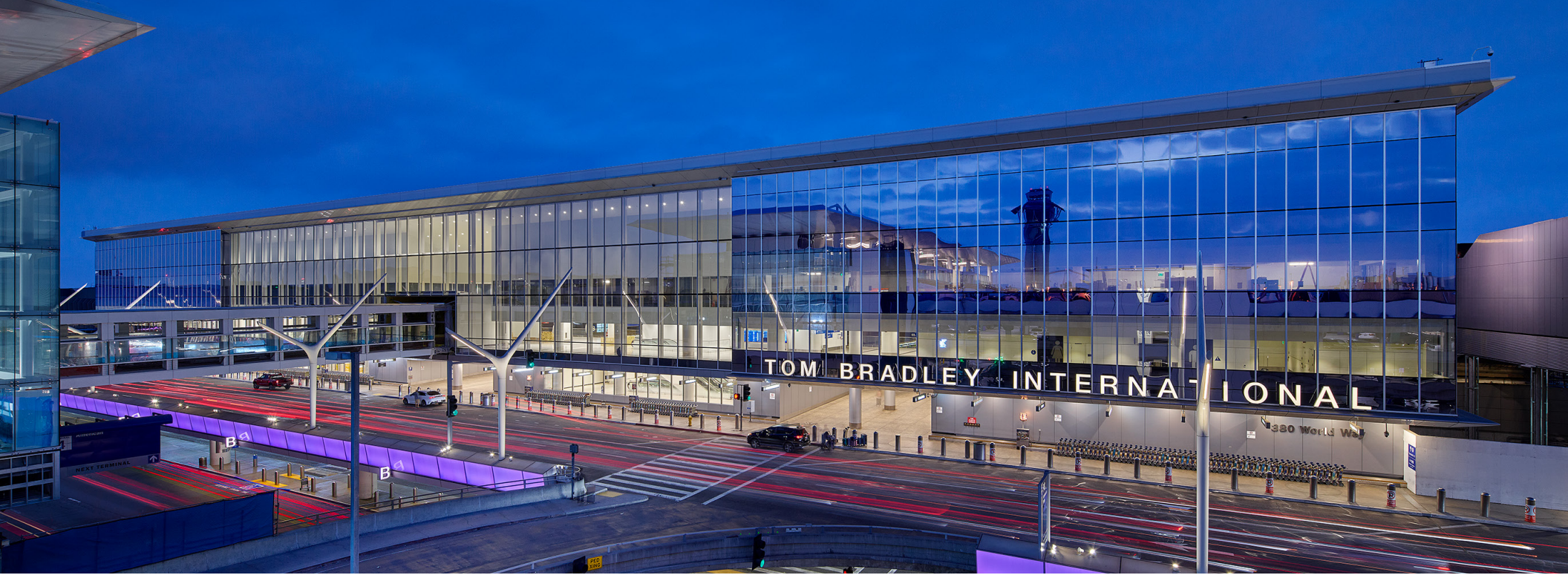
LAX Vertical Circulation Cores, LEED Silver
