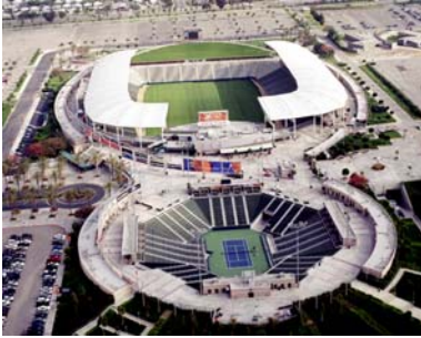
Home Depot Center
