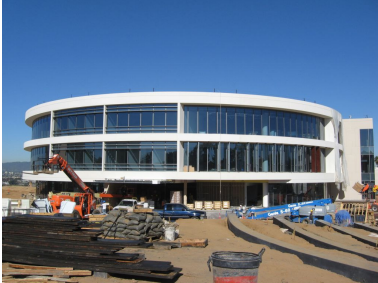
Caltrans District 7 Headquarters
